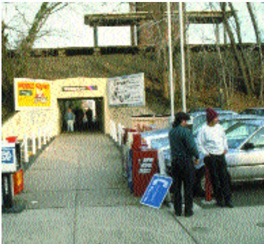
Before - Pearl Street Entrance, NJ Transit Woodbridge Train Station
