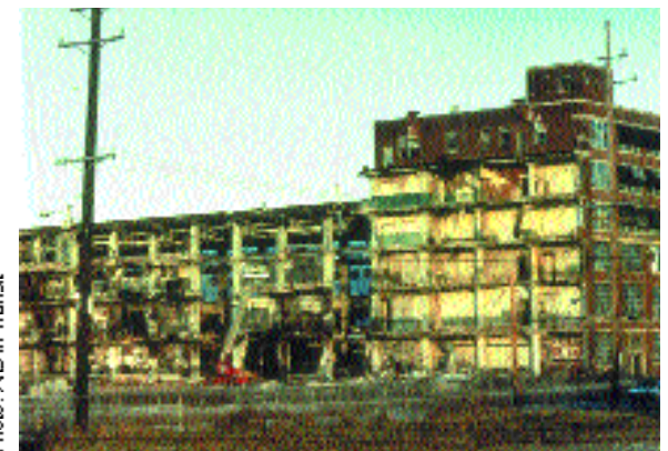
Wagner Electric Factory - Before
