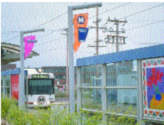
Wellston MetroLink Platform
